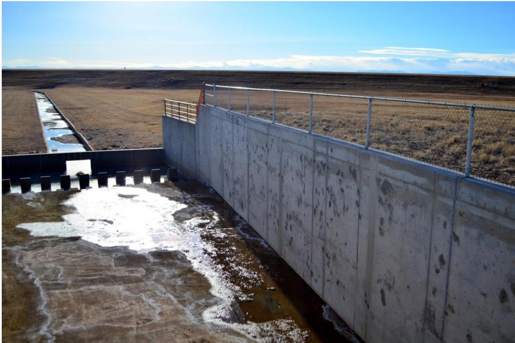
**Figure 6.1.** Box culvert at DIA receiving stormwater runoff from the west side of the airfield.
