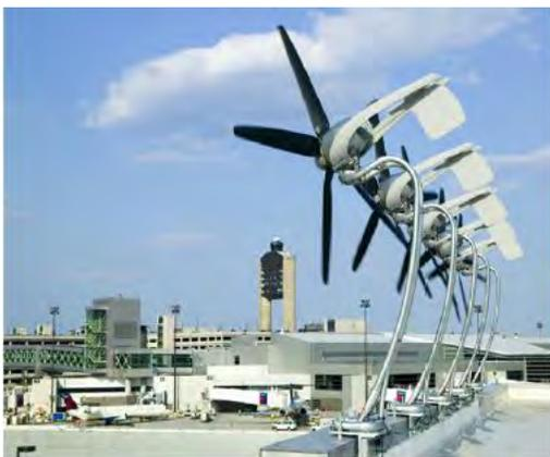
Although not mounted on a JBF, AeroVironment has already partnered with BOS airport and installed twenty Architectural Wind turbines on top of one of the airport’s buildings (Ritchie, 2009).
